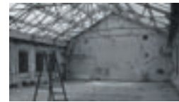
PIARISTEN- GASSE 17 Co-Working Space Wien
